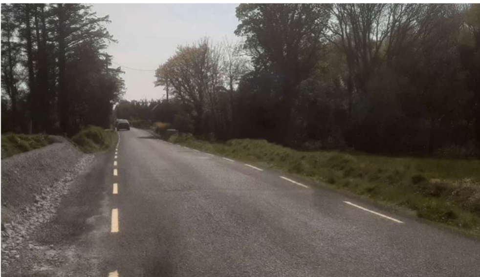
Image 1.7: Example of a Reinstated Road Following the Laying of Underground Cables
