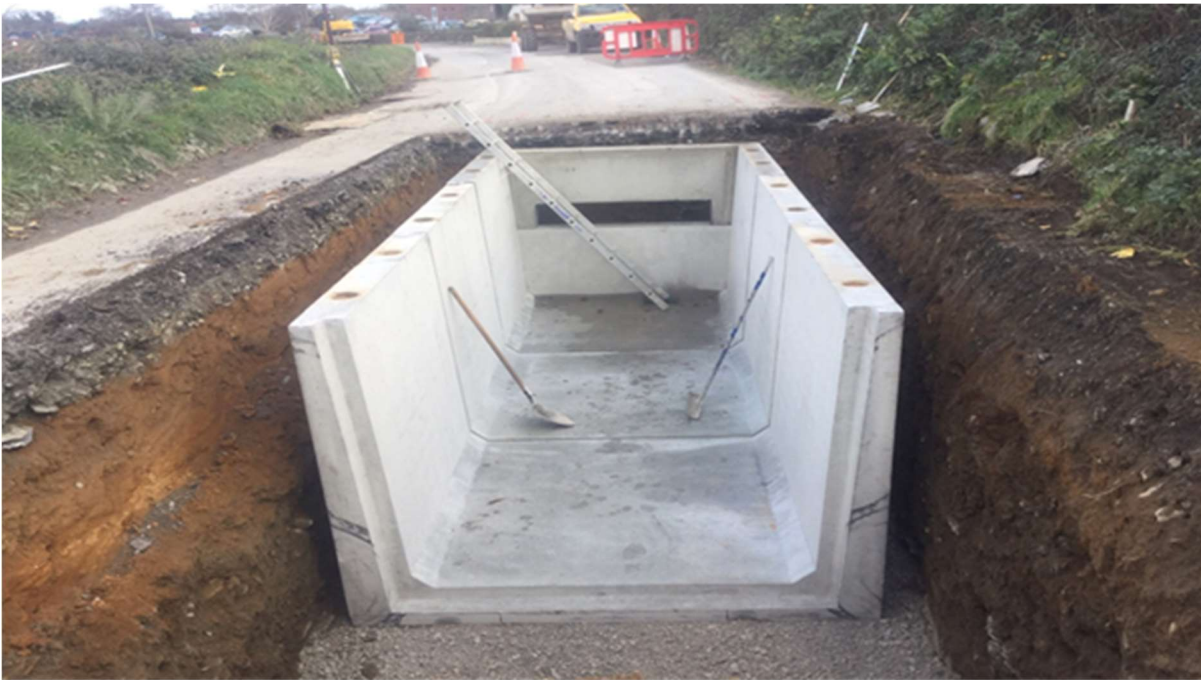
Image 1.3: Example of a Joint Bay During Construction
